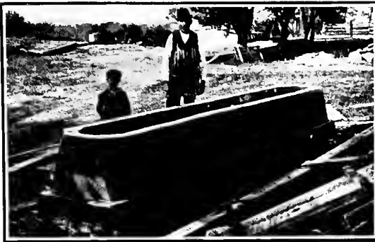
FIG. 222—CEMENT WATERING TROUGH.
